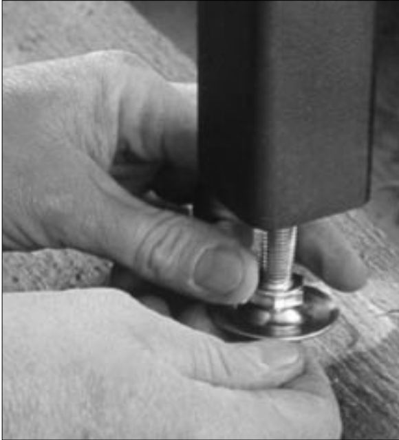
Fig 6 Fit the 4 adjustable feet before you lift the hearth unit off the pallet.
