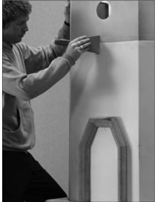
25. Apply filler (included in the delivery consignment) between the metal extension cover and the casing.
