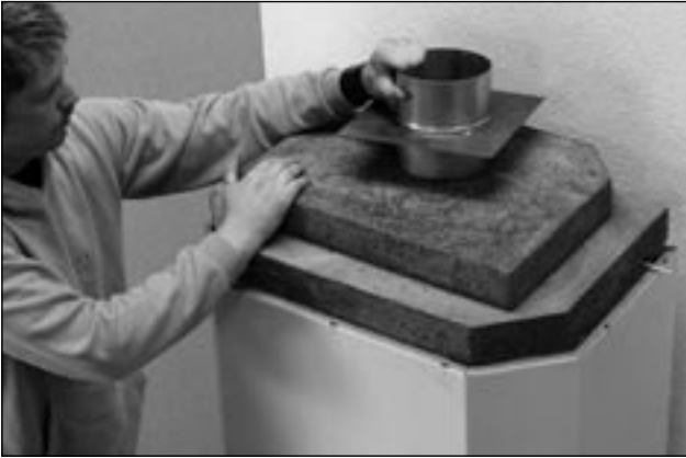
13. If a steel chimney is to be used, a connection insert is normally required. Smear a thin layer of stove sealant onto the insert and push it down into the top element. N.B. The connection insert is included in the chimney delivery, and should be specified when placing the order.
