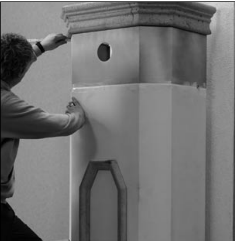
26. Lift the canopy/crown into place, check that it is properly centred and attach it with silicon adhesive.
